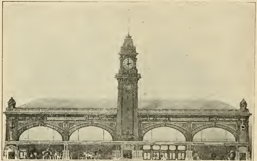
NEW FERRY HOUSE—NEW YORK TERMINAL OF THE LACKAWANNA.
